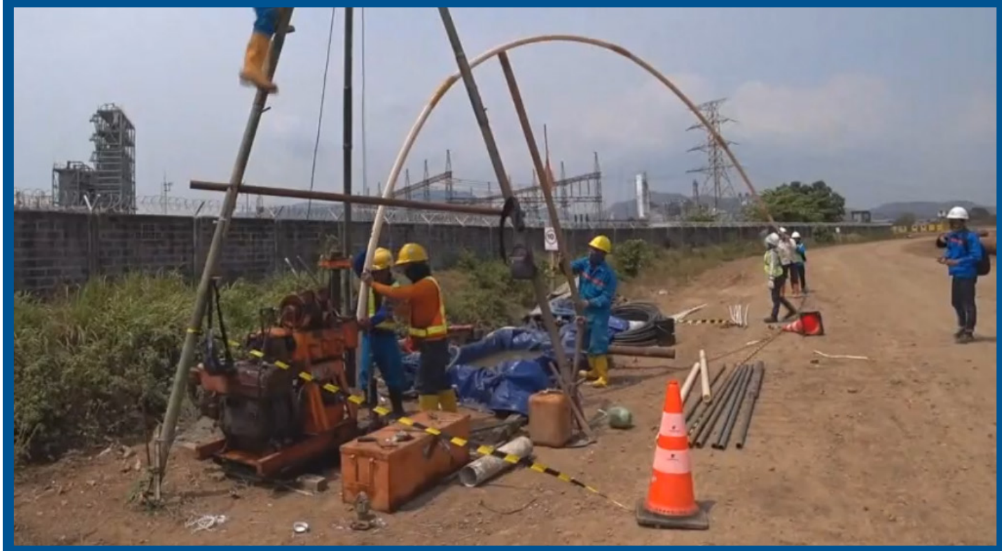
Workers installing the inclinometer tube
